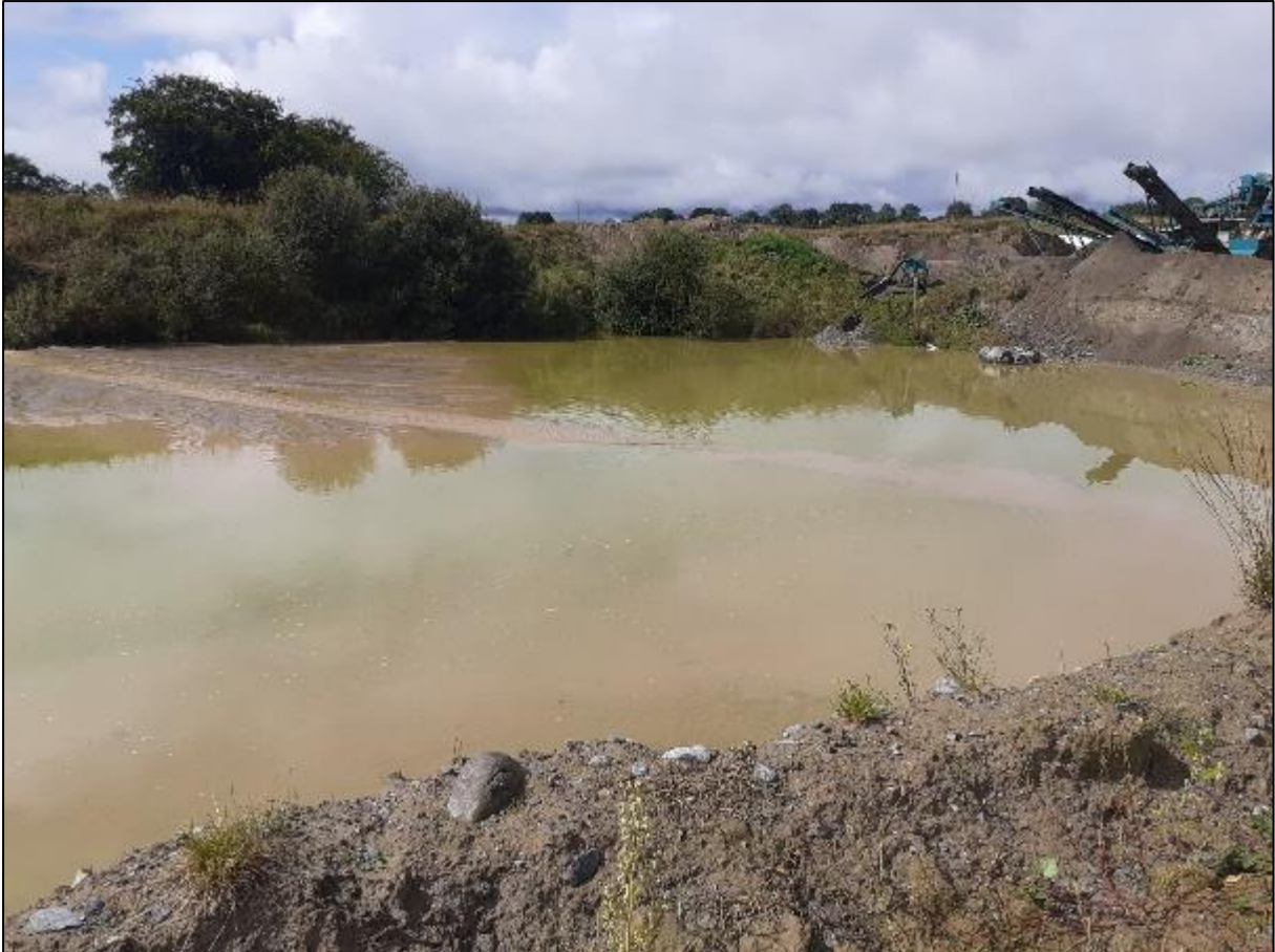
Figure 5-10: Extraction/settling pond located within the active quarry
